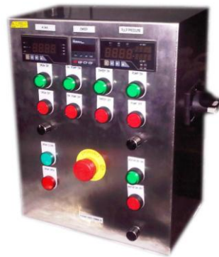
Control Panel with 3 digital displays
